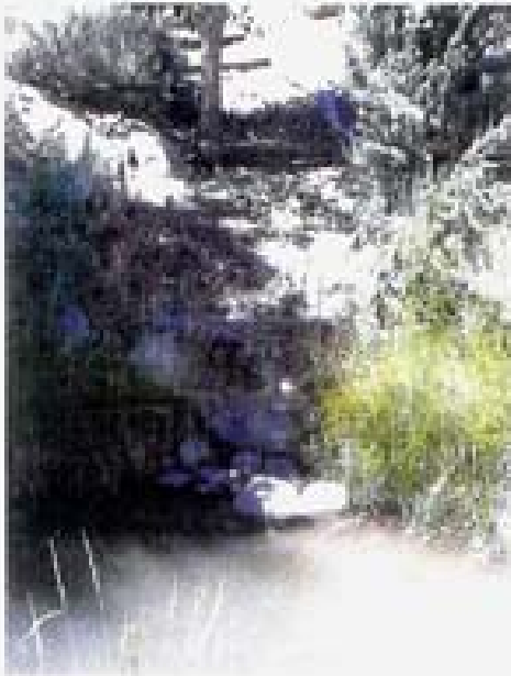
Point 42. Small drainage swale allowing backyard runoff to enter the Steamboat Ditch.
