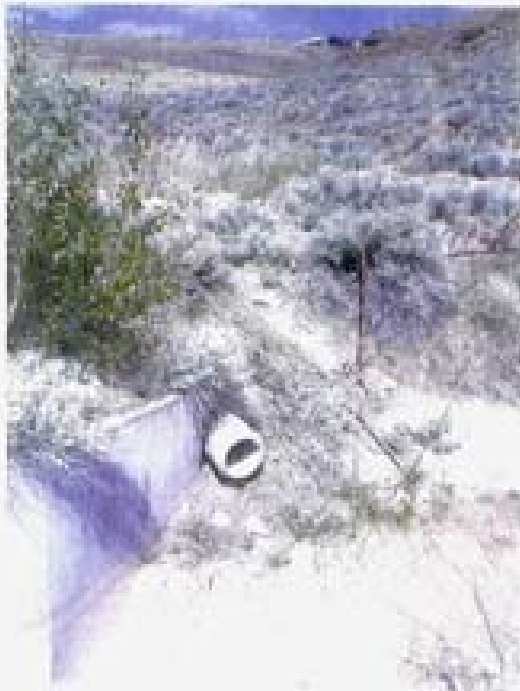
Point 14. A 12" I.D. concrete pipe empties into the Steamboat Ditch at the box culvert at Anitra Drive.
