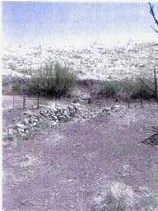
Point 25. A small rip rap lined drainage allows water to exit the Steamboat Ditch. In addition, a sluice gate is located a few meters downstream of the larger gate structure.
