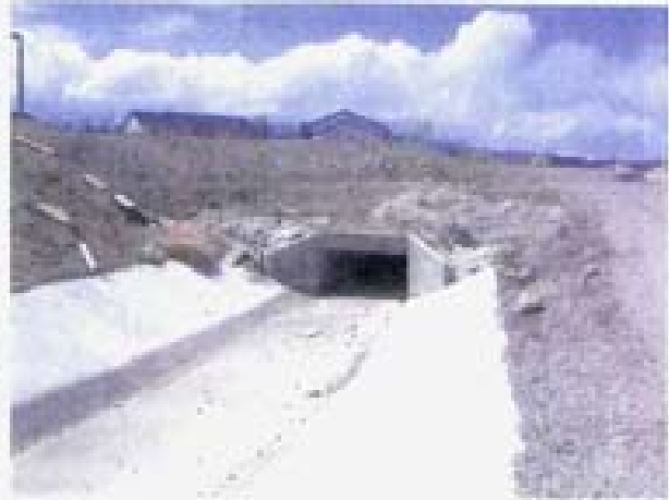
Point 50,51. Box culvert crossing under Wedge Parkway and under the flood conveyance structure from Whites Creek.
