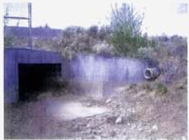
Point 14. A 12" I.D. concrete pipe empties into the Steamboat Ditch at the box culvert at Anitra Drive.
