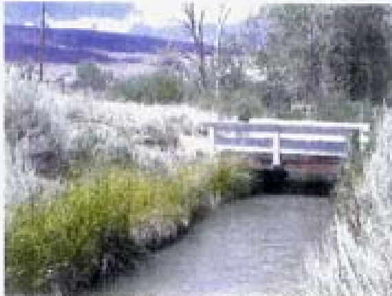
Point 35. Bridge crossing near Fricke Lane.
