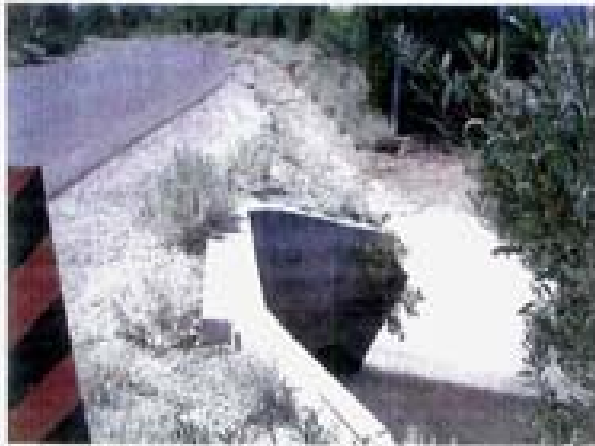
Point 40. Small swale carrying drainage waters from Oak Glen Drive (near Zolezzi Lane) into the Steamboat Ditch.
