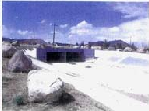
Point 51 cont. View of Steamboat Ditch to the right and the flood conveyance channel for Whites Creek to the left. The photo on the right shows the double box culvert for flows from Whites Creek crossing under Wedge Parkway.
