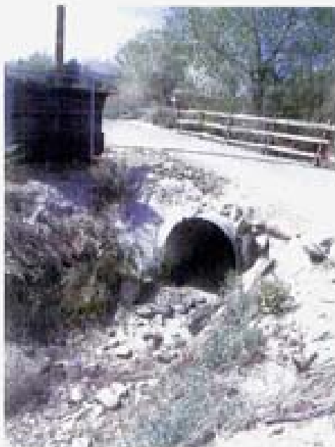
Point 49. Steamboat Ditch crosses under a one-lane private road through a large CMP pipe. Note the concrete swale funneling stormwater runoff to the ditch. The photo on the right shows erosion along the roadside where stormwater has entered the ditch.
