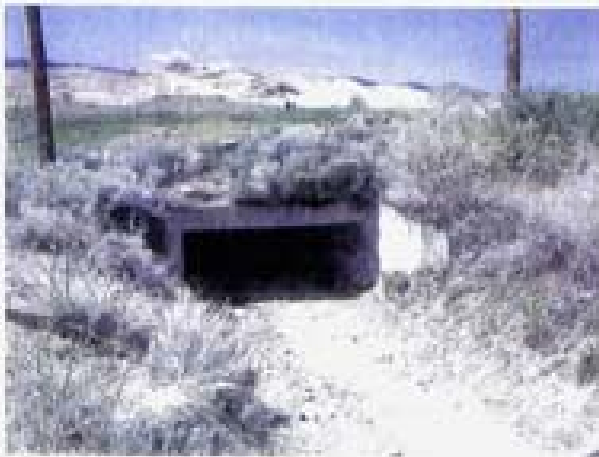
Point 20. Box culvert on Bell Haven Road where the Steamboat Ditch crosses under the road.
