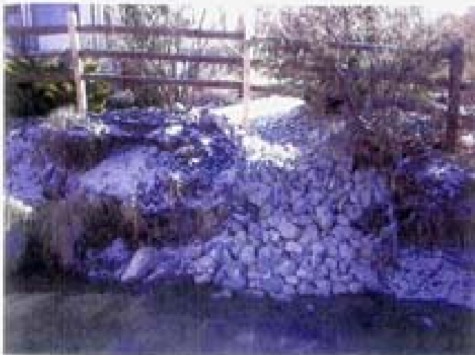
Point 6. Small rock lined swale discharging from a private parcel.
