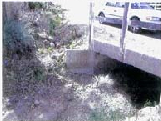
Point 29. Box culvert where Lamay Lane crosses the Steamboat Ditch. Drainage swales along both sides of the road carry discharge into the Steamboat Ditch.
