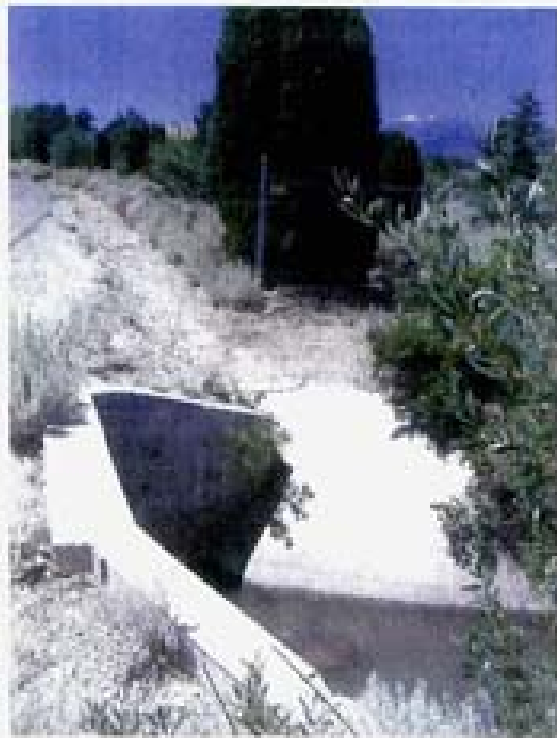
Point 40. Small swale carrying drainage waters from Oak Glen Drive (near Zolezzi Lane) into the Steamboat Ditch.
