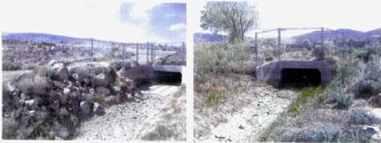
Point 48. Box culvert crossing under Arrow Creek Parkway.
