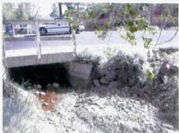
Point 29. Box culvert where Lamay Lane crosses the Steamboat Ditch. Drainage swales along both sides of the road carry discharge into the Steamboat Ditch.
