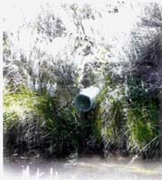
Point 37. Small green plastic/PVC pipe draining a private parcel close to the cul-de-sac at Thomas Creek Drive.
