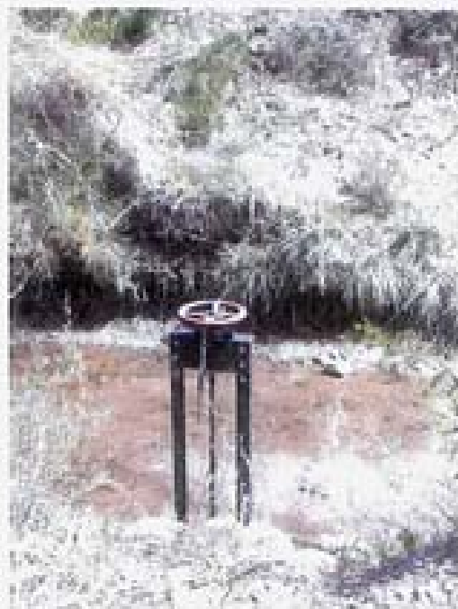
Point 25. A small rip rap lined drainage allows water to exit the Steamboat Ditch. In addition, a sluice gate is located a few meters downstream of the larger gate structure.
